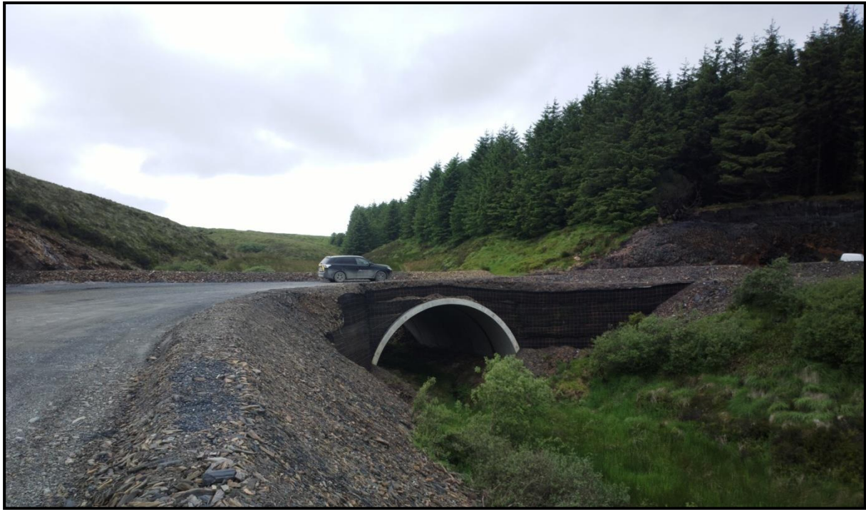
Figure 4-8 – Completed clear span pre-cast concrete culvert crossing over an existing watercourse
