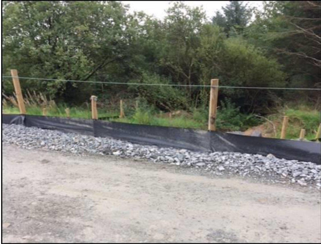
Figure 4-5 – Dirty water containment at watercourse crossing
