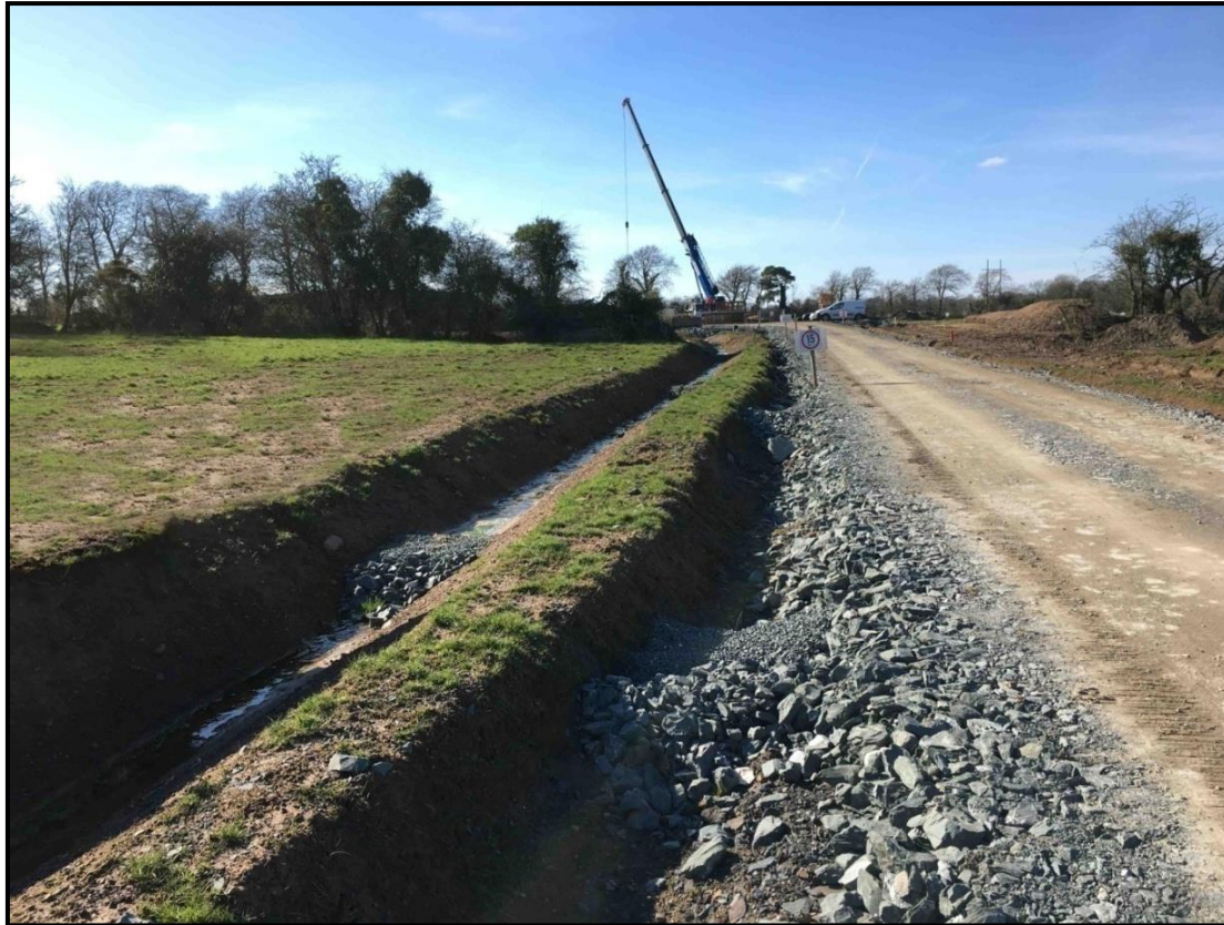
Figure 3-1 – Separation of clean and dirty water drainage on a wind farm site
