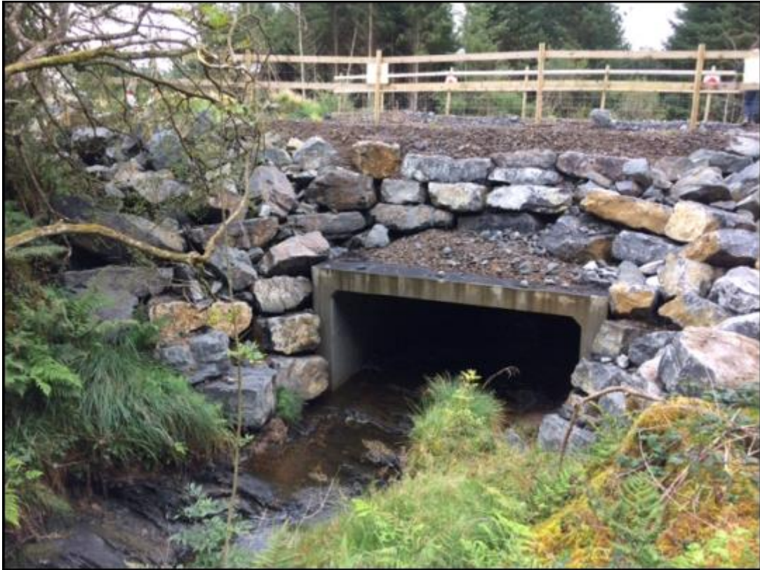
Figure 4-4 – Typical drainage channel crossing
