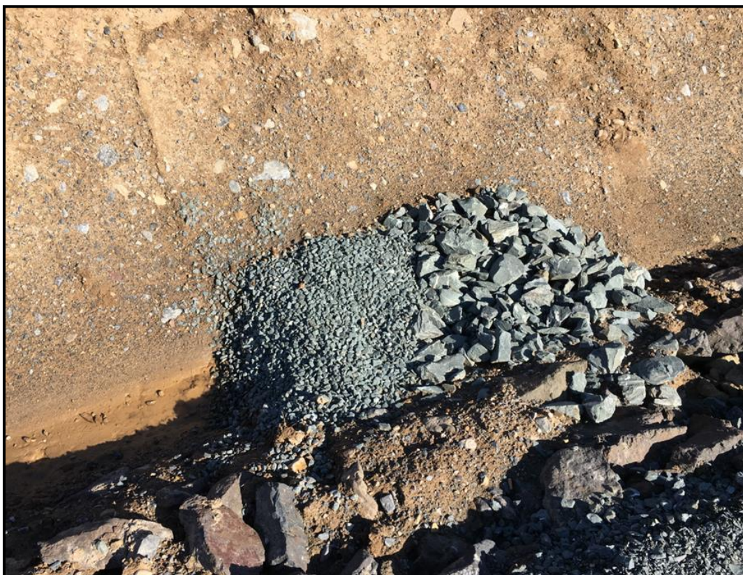
Figure 3-3 – Stone check dam with large aggregate on downstream side
