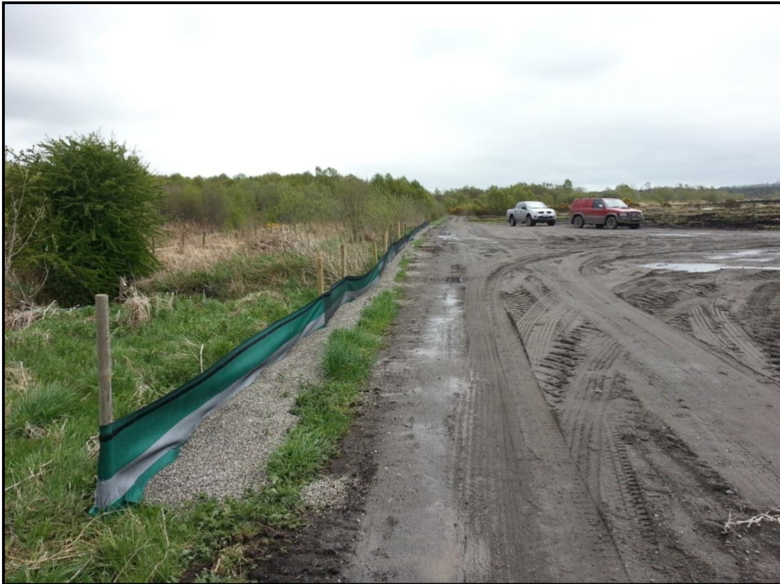
Figure 4-6 – Silt curtain containment along existing roads near watercourses
