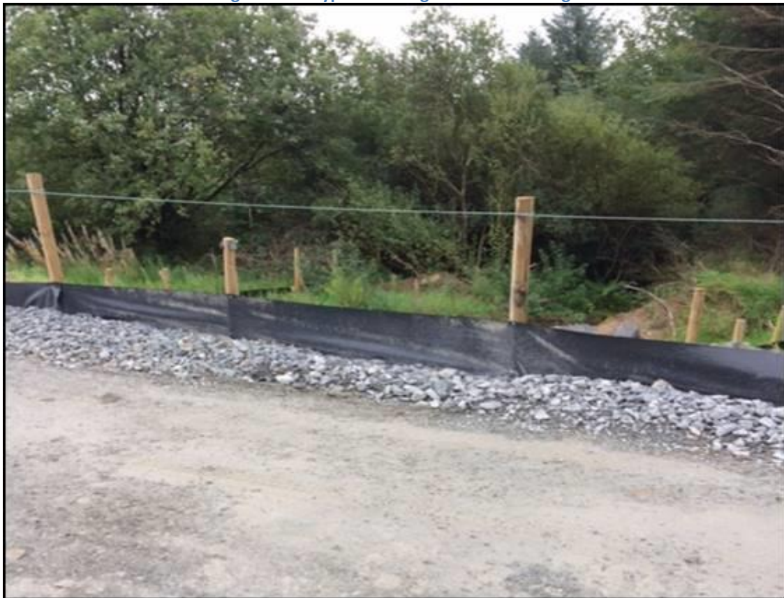
Figure 4-4 – Typical drainage channel crossing
